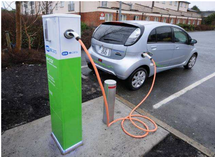
Figure 2.1 - AC Charge Point
