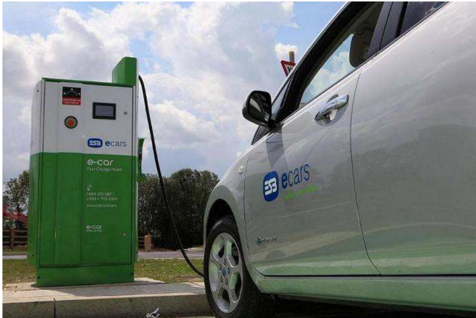
Figure 2.2 - DC Charge Point
