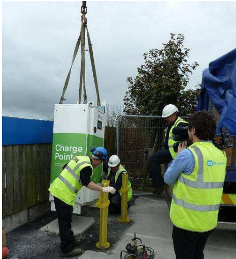
Figure 4.20 - Installation of DC Fast Charge Point using HIAB
