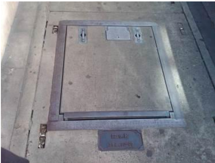
Figure 4.13 - Underground Vault in Paris
