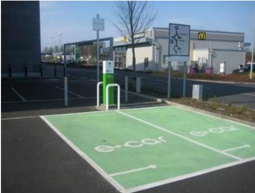
Figure 4.1 - Charge Point in Shopping Centre Carpark
