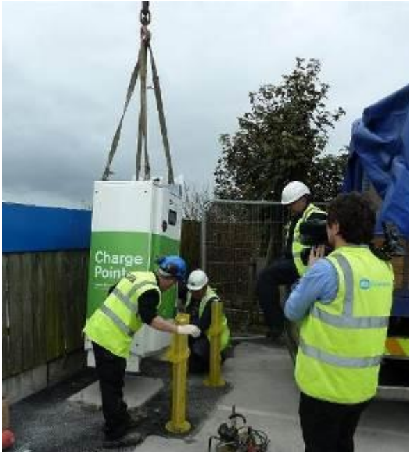
Figure 4.21 - Installation of DC Fast Charge Point using HIAB
